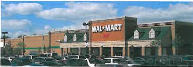
Design standards can improve the appearance of the building and site landscaping, but are not effective in changing the underlying form.
