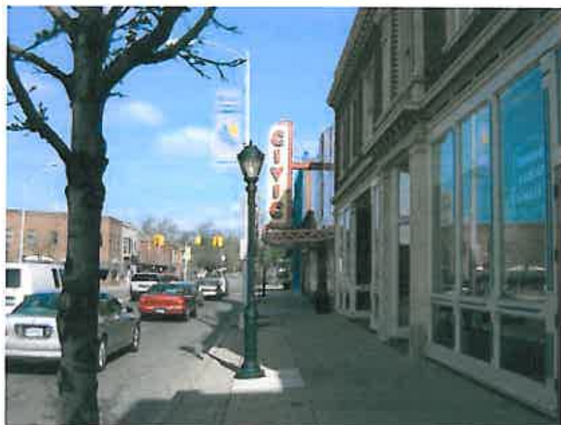
Farmington has adopted a form-based code as part of the central business district that reflects the traditional urban fabric that the community values.
